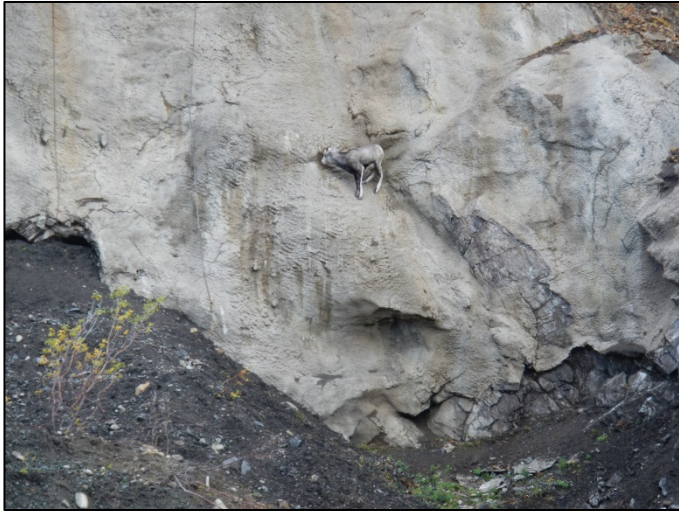
Photo 3. 1465 Portal. Note sheep on shockcrete.
