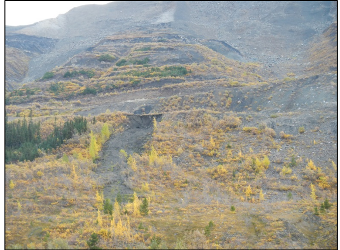
Photo 6. Slump above 1465 Portal
